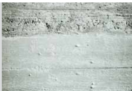
Grout applied by brush, coarse board formwork texture maintained
