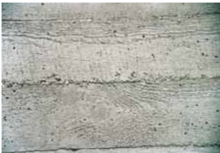
Mineral stain finish (without filler), pores and cavities remain open
