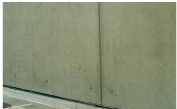
Blemishes largely toned down with KEIM Concretal-Lasur
